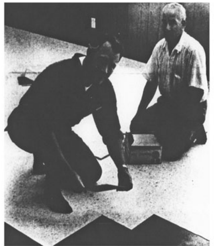
LAYING FLOOR IN NEW CATHOLIC SCHOOL
