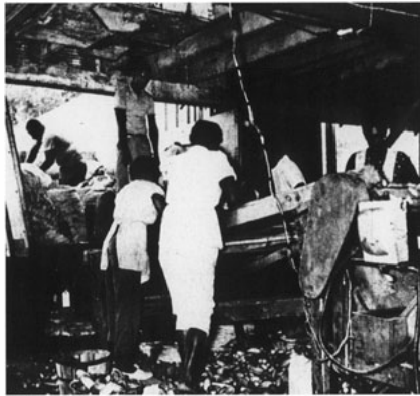
SWAFCA GRADING STATION
