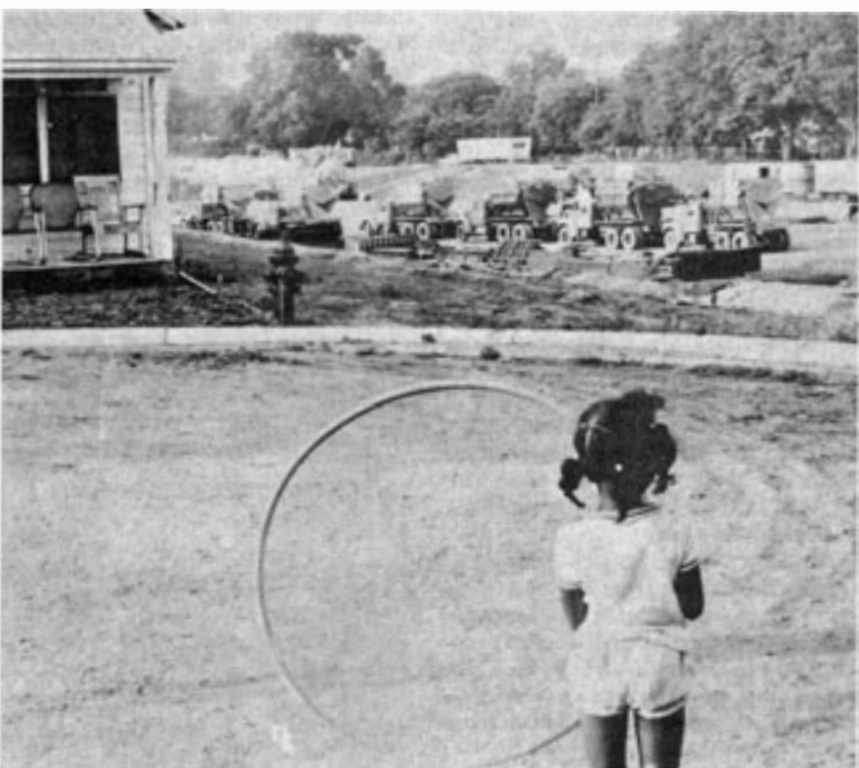
SITE OF NEW INTERSTATE HIGHWAY
