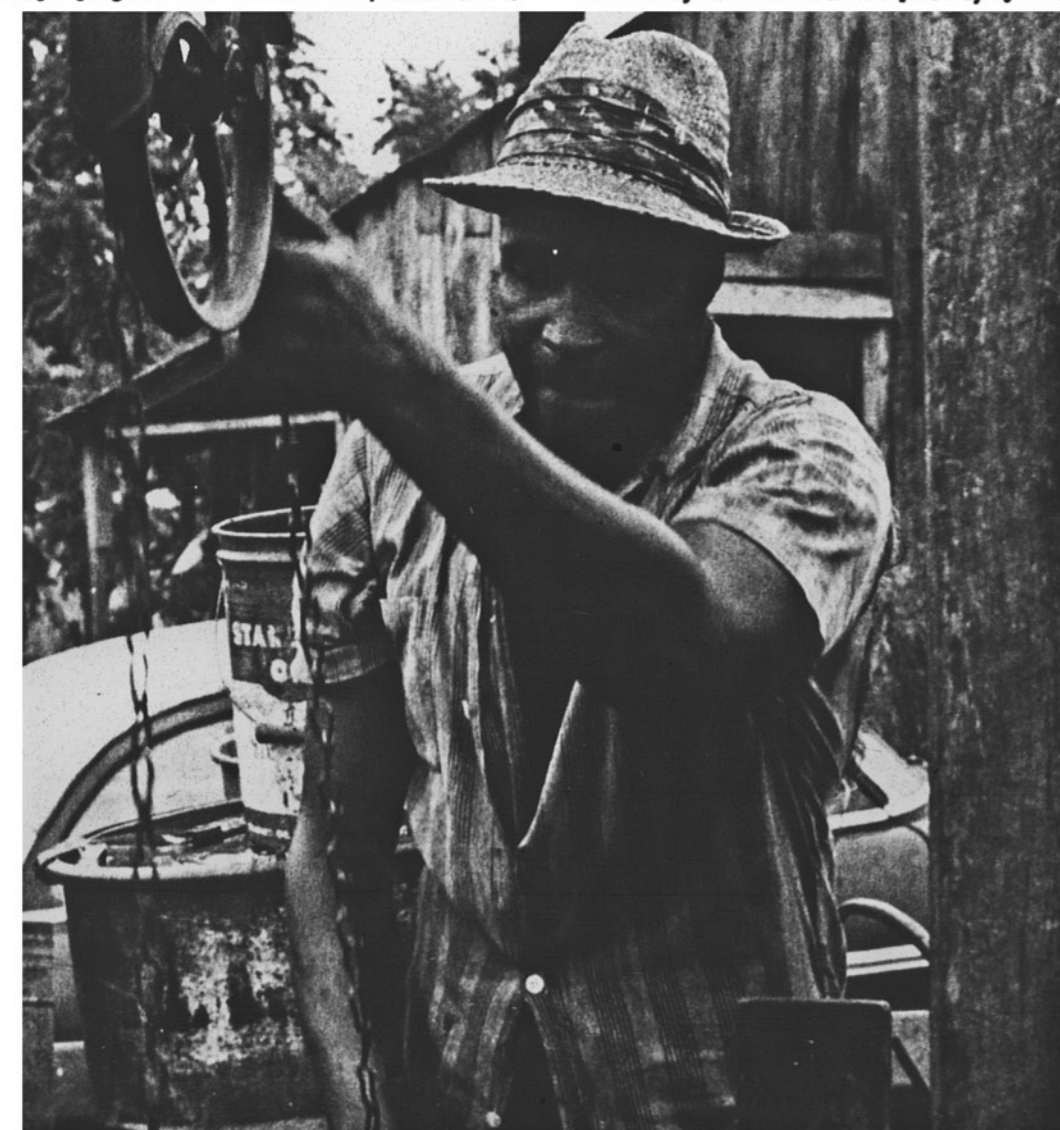
TRIANA RESIDENT DRAWS WATER FROM WELL. PIPES WILL BE LAID THIS FALL.
