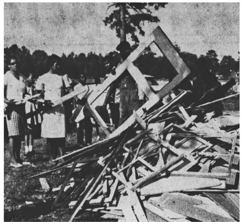
AFTER MYSTERIOUS BOMBING LAST MAY, CHURCH MEMBERS WERE LEFT WITH ONLY WRECKAGE--AND A WILL TO REBUILD LOST CHURCH BUILDING.
