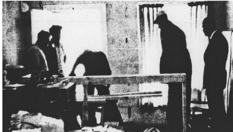
REMODELING THE OFFICE
