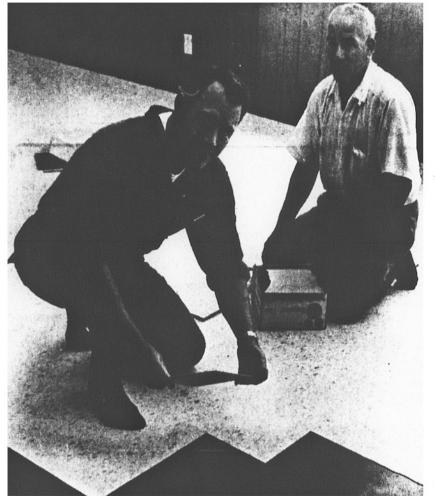
LAYING FLOOR IN NEW CATHOLIC SCHOOL
