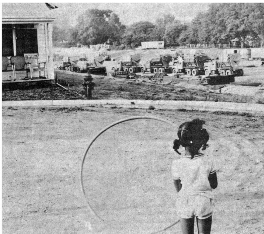
SITE OF NEW INTERSTATE HIGHWAY
