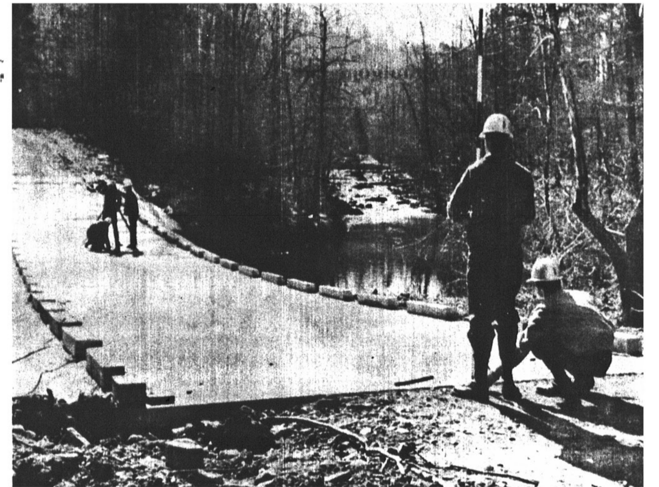
JOB CORPSMEN SURVEY ROAD IN ARKANSAS
