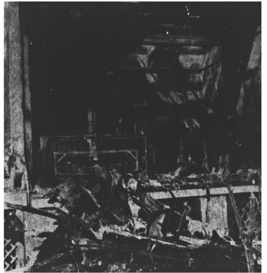
BURNED HOME ON SOUTH WARREN STREET
